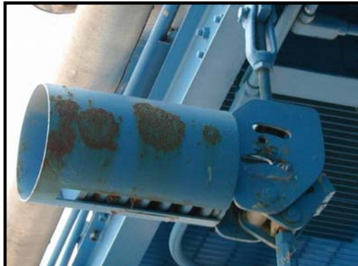
Figure 1. Constant Support Hanger Fouled by Nesting Birds
