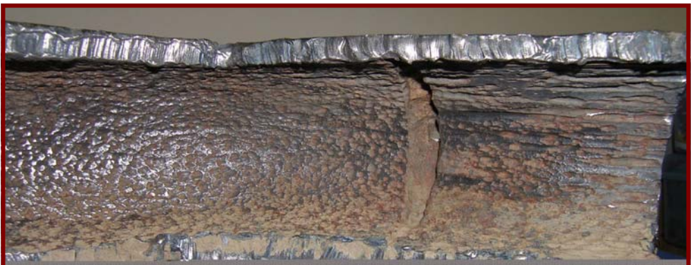
Figure 1. OTSG return pass bend (longitudinal section) showing typical single-phase FAC “orange peel”, along with grooves (merged pits).
