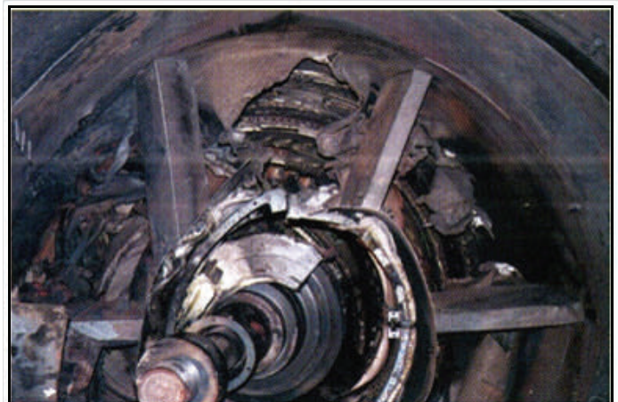
Figure 1. Power turbine failure exhibits considerable collateral damage.
